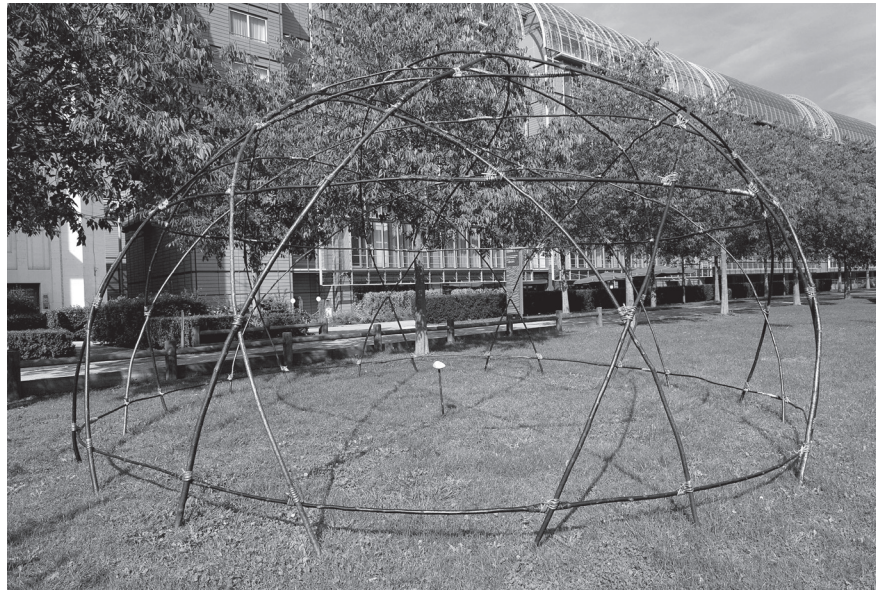
Great Circle Dome, 1960 Bois de châtaignier et noisetier, Ø 6m Courtesy The Estate of R. Buckminster Fuller Collection mac LYON © photo Blaise Adilon
