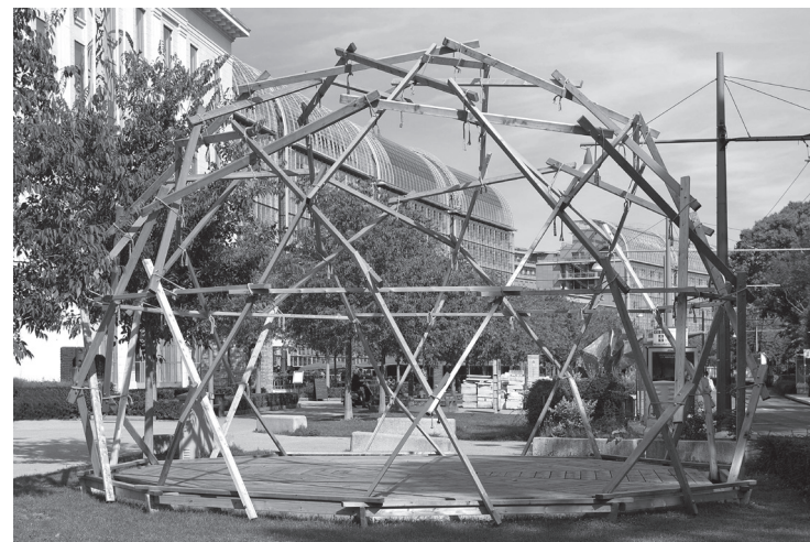
Bear Island Dome, 1965 Bois de mélèze, Ø9m, Courtesy The Estate of R. Buckminster Fuller Collection mac LYON © photo Blaise Adilon
