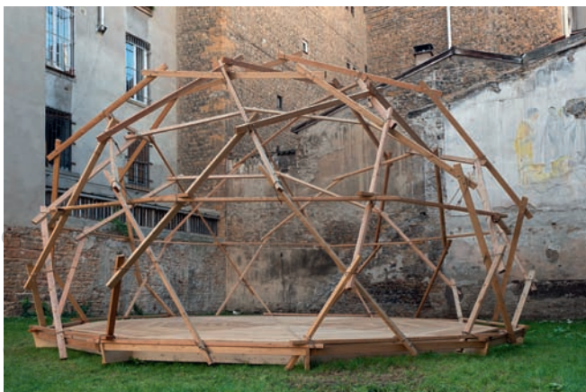
Richard BUCKMINSTER FULLER, Bear Island Dome , 1965 Bois de mélèze, Ø 9m Biennale de Lyon 2011, Courtesy The Estate of R. Buckminster Fuller Collection mac LYON © photo Blaise Adilon
