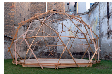
Bear Island Dome Conception 1965, reconstruction 2004, construction in Lyon 2011/2012 Larch wood, 9m diameter, Designed by Fuller rebuilt under Deacon Marval's supervision © Blaise Adillon
